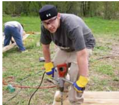
Brad building lunkers
