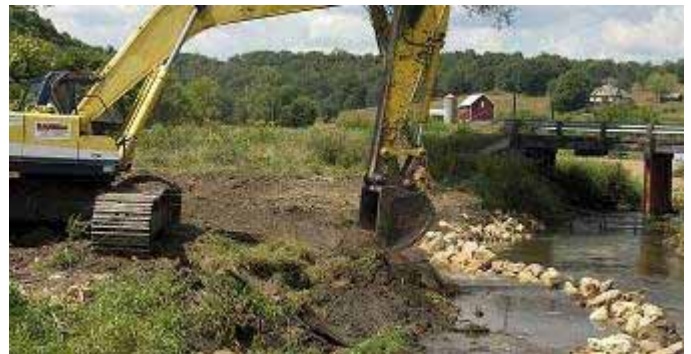
Filling in behind the rocks of a now-narrowed stream section.
