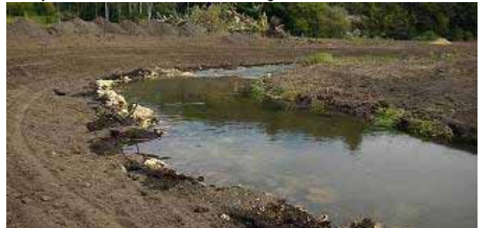
The same bend leveled and stabilized with rock.
