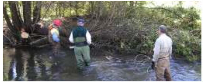
A hearty crew installs a sweeper
